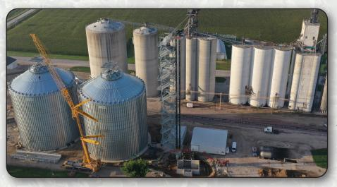
The bins are fully erected! We are so excited to finally see almost fully constructed grain bins. The construction crew still needs to put the catwalk in above the bins, the conveyors, etc. They are also pouring the last portion of the bootpit. Photos from the morning of 8.23.2023. More updates coming soon, there will be lots of exciting developments within the next 20 days as we approach harvest! The plan is still for the project to be ready to dump grain this fall.
