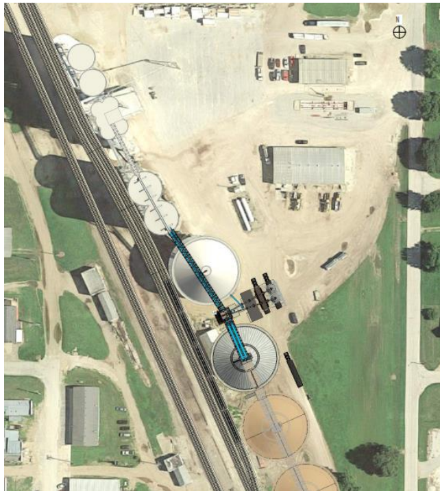
The photo above is detailing an overhead photo of the new bin that is to be constructed in Graettinger as well as the new overhead load out.
